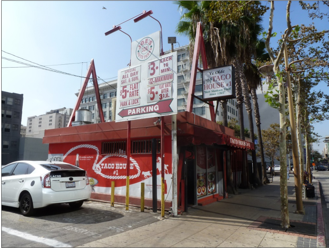
Figure 4: Southeast view of the building at 342 South Hill Street. Source: GPA
